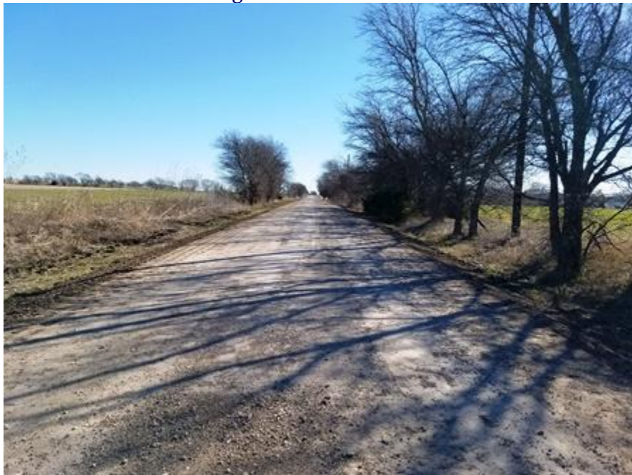
Recycling process of Chisum Road.
