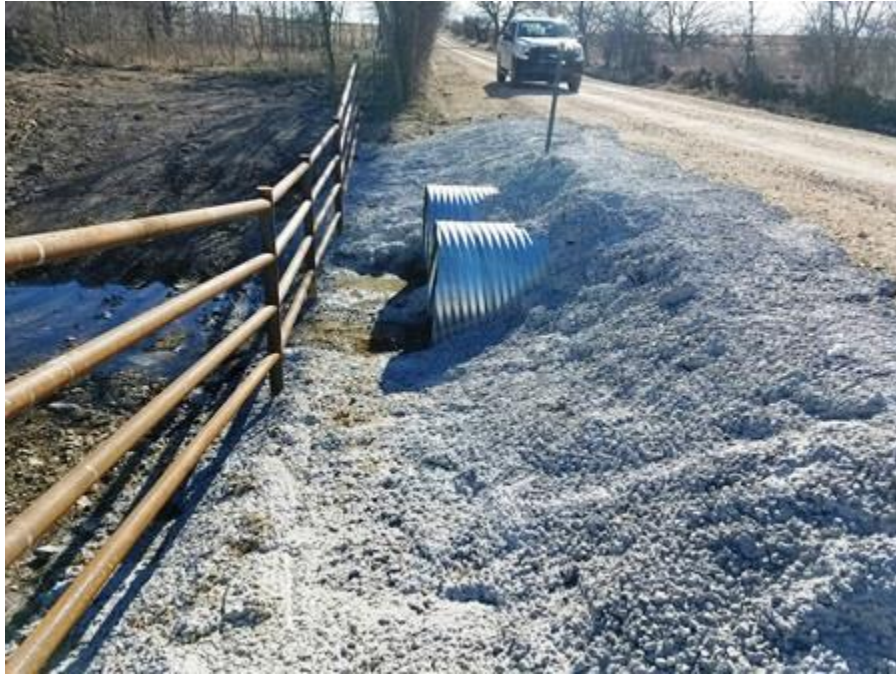
Concrete rip-rap on Waide Road.
