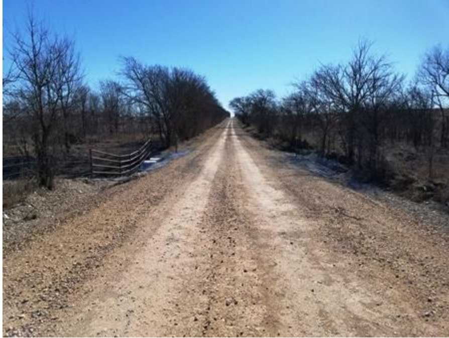
Completed drainage work on Waide Road.
