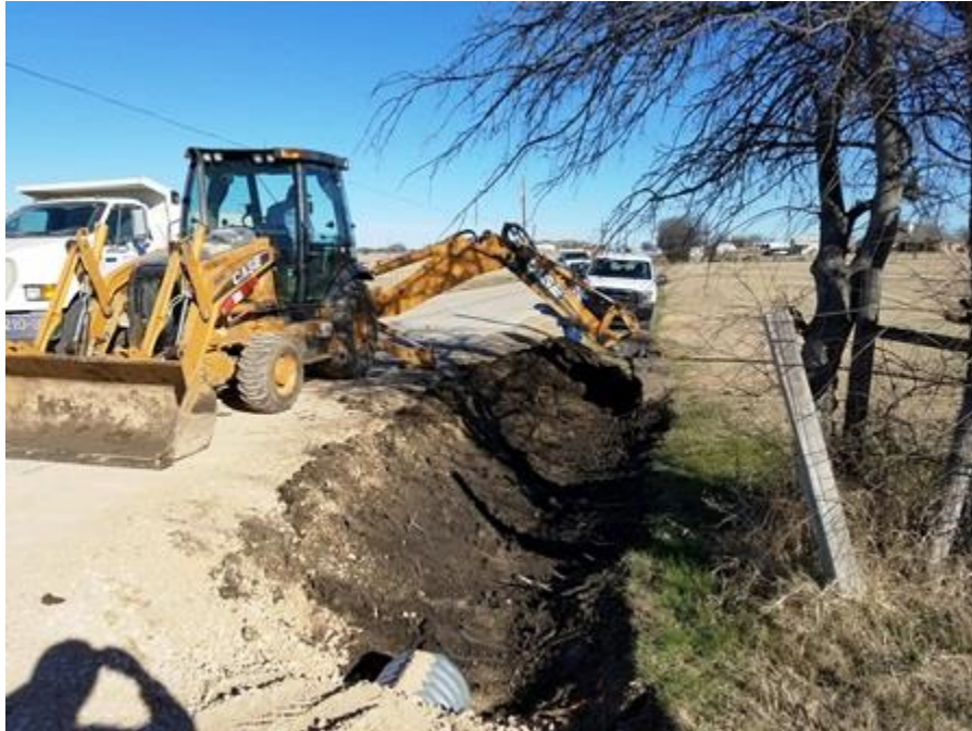
Drainage work on Chisum Road.
