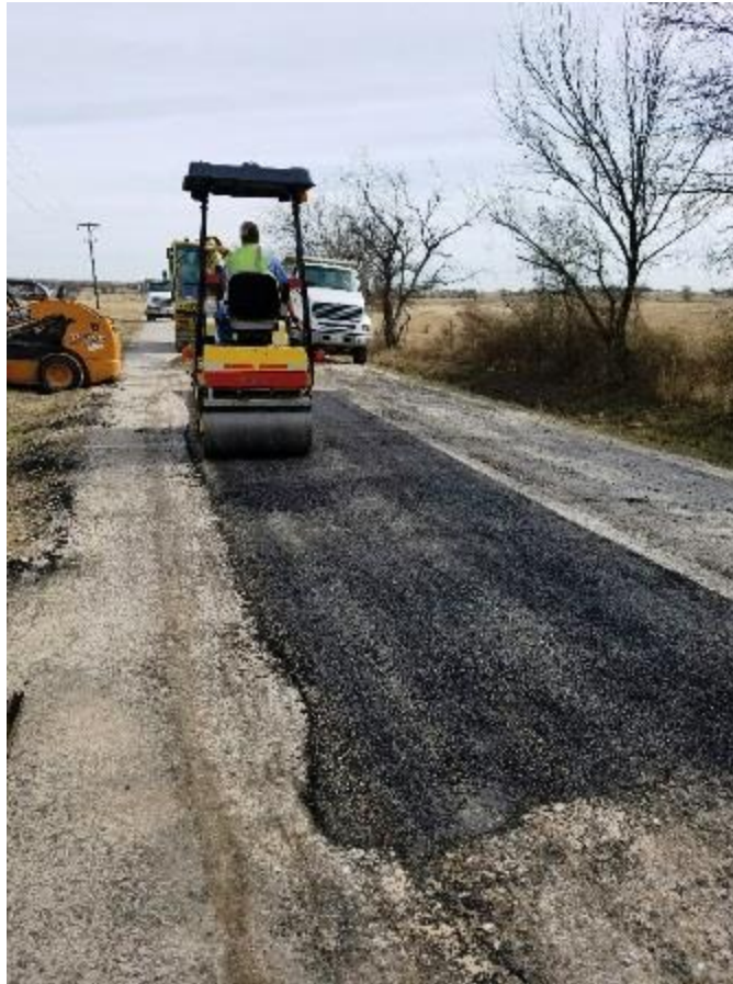
Repairing base failures on Michael Road.
