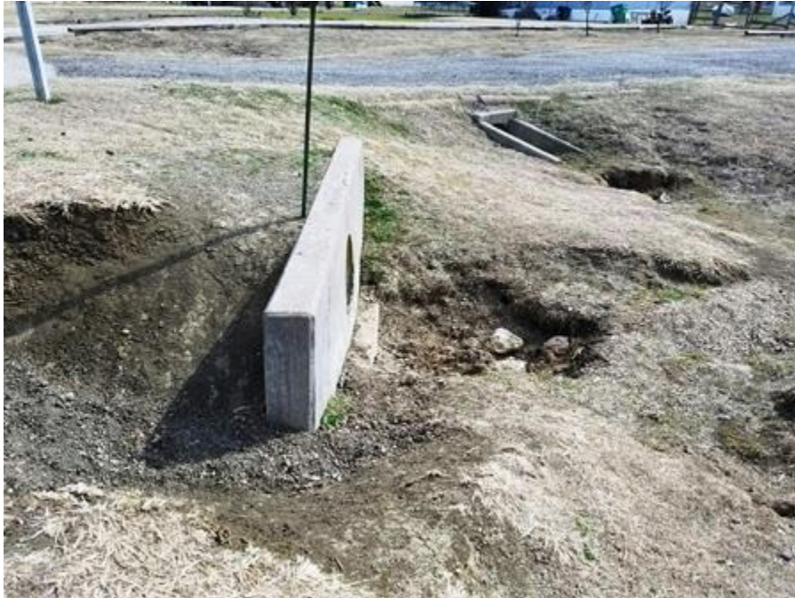
Addition to concrete head wall on Meadow Vista Circle.
