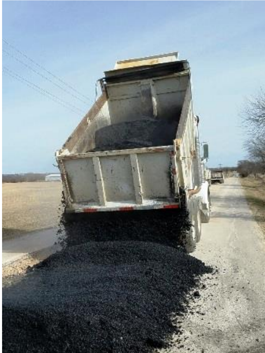
Repairing base failures on Michael Road.
