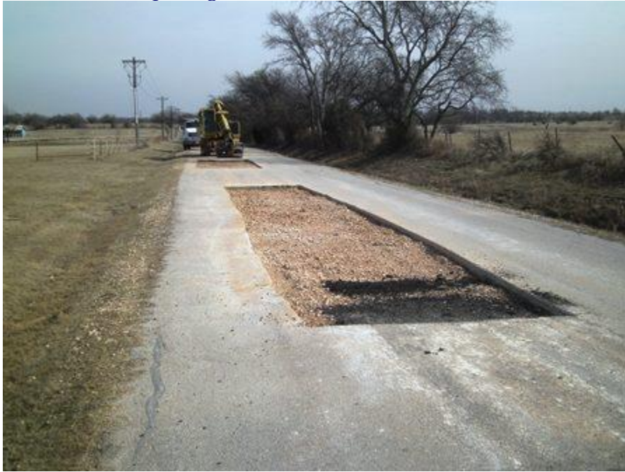
Repairing base failures on Michael Road.
